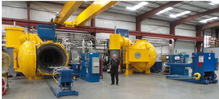
Pictured: Chuck Miller, Maintenance Manager/Facilities Engineer at the Solar Atmospheres California facility, who managed the building and support systems design and fabrication along with the new equipment design and installation.
